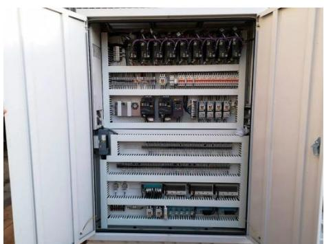
A sealed dust- and moisture-resistant cabinet with electronic components from the world's leading manufacturers is removed from the processing area, which extends the service life of electrical components and ensures ease of maintenance
